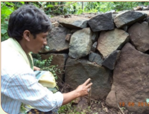
Installation of erosion pins on U/S of LBCD
